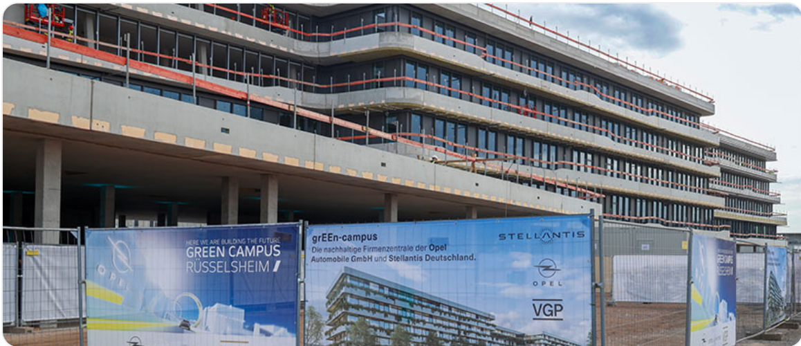
Bauschild GREEN CAMPUS
